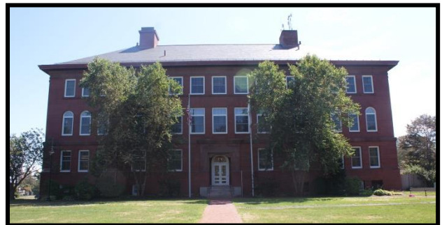
Town Hall Renovations, 2010
